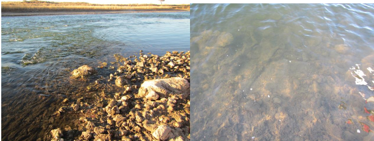
Figure A.3.2. Site 1 - Morad Park, standing on right bank, looking across the channel at Rock vane 1 (left). The header boulders are visible above base flow in the foreground (left). Boulders underwater at the same level of the surrounding substrate further into the channel (right).
