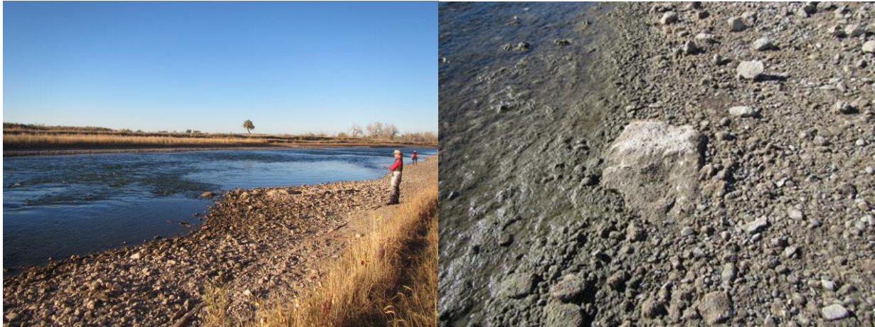
Figure A.3.1. Site 1 - Morad Park, standing on the left bank, looking downstream at the constructed riffle (left) on 10/15/2018. Arm 1 of the constructed riffle is in the foreground, with multiple boulders visible out of water on the right bank. Turbulence from arms 2 and 3 can be seen downstream in background. On the left is one of the only visible boulders in the fourth (most downstream) arm of the constructed riffle.
